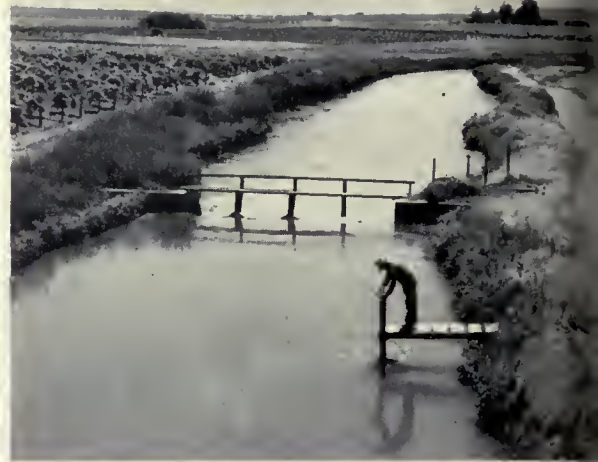
BEWARE OF THE VACUUM! —At left, note the rectangular opening in front of the pipes. When water in Colorado-Big Thompson Horsetooth Feeder Canal rises above normal, the siphon spillway goes into automatic operation, and a vacuum, strong enough to suck a man into the spillway, is created. Above, currents around check structures (like this one on the Sunnyside Canal Yokimo project, Wash.) are extremely dangerous. Photo of left by A. E. Thompson, above by S. T. Larsen.
